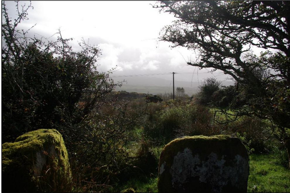
Photograph 5 - View of the Pole 63 of the constructed OHL
