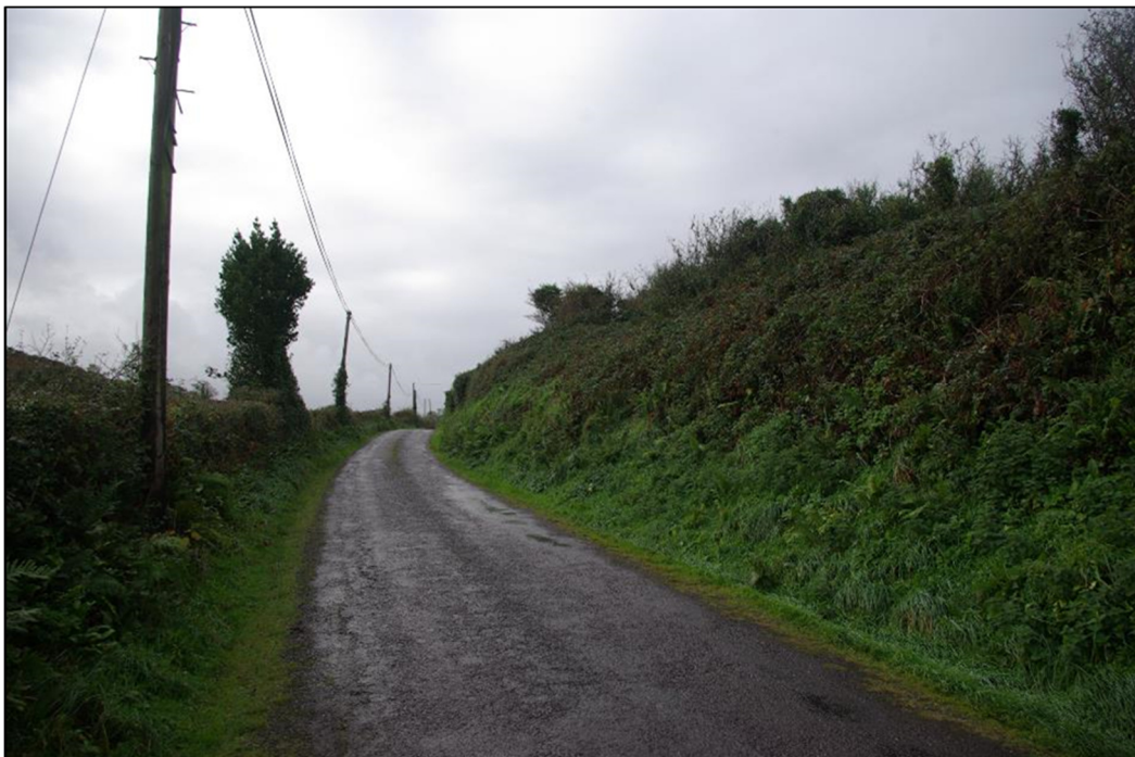
Photograph 5: View south-westwards along the section of roadway in Shandrum Beg townland where underground cabling is proposed to extend.
