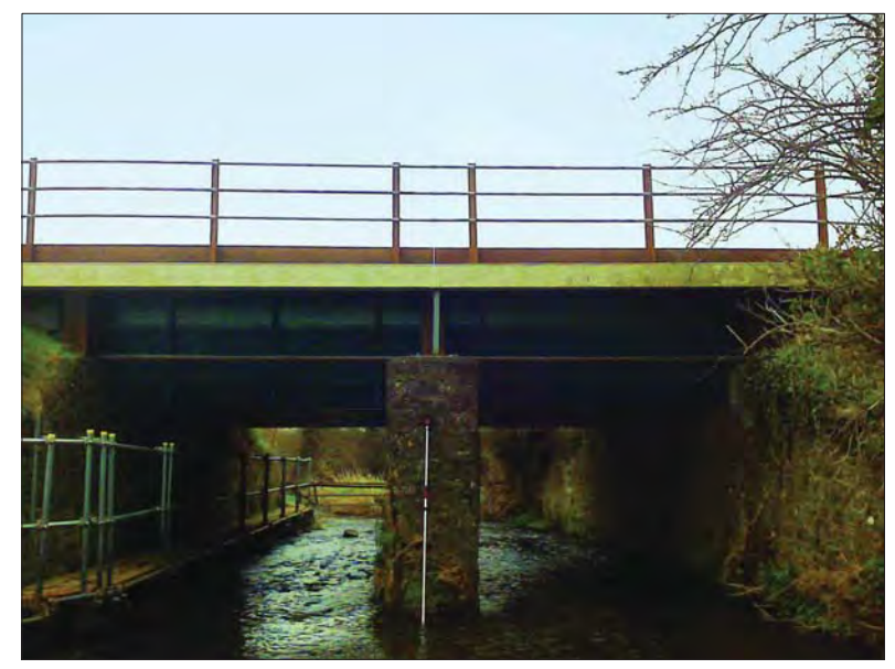
PHOTO VIEW 1 - Existing Bridge at Painestown River / Culvert No. 10, Painestown (Not to Scale - Downstream View)
