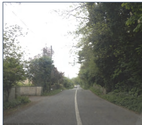
Image 6.14: L6021 Fingerpost Bridge
