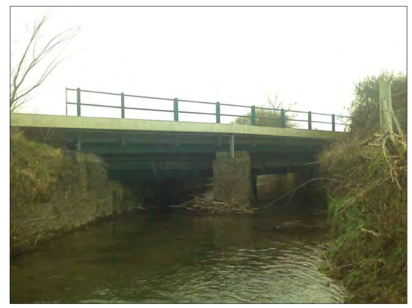
RAIL BRIDGE OVER RIVER MORELL (DOWNSTREAM)
