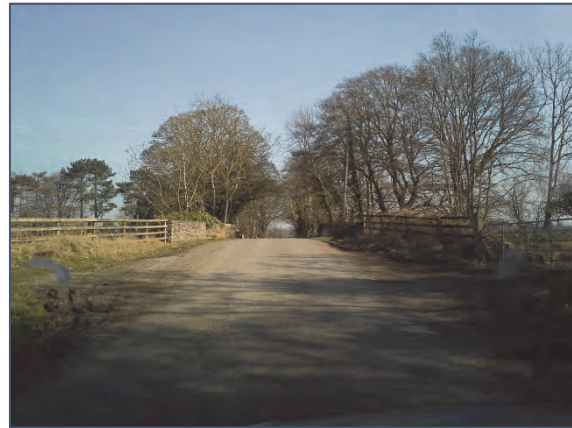
Image 6.6: Morell Bridge (old) on L6016
