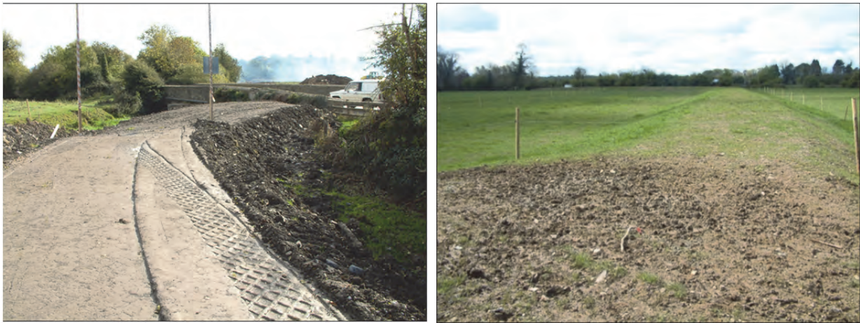
Image 4.1: Example of an Embankment During Construction
