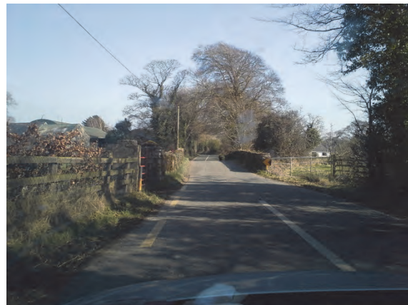
Image 6.12: L2010 Painestown Bridge
