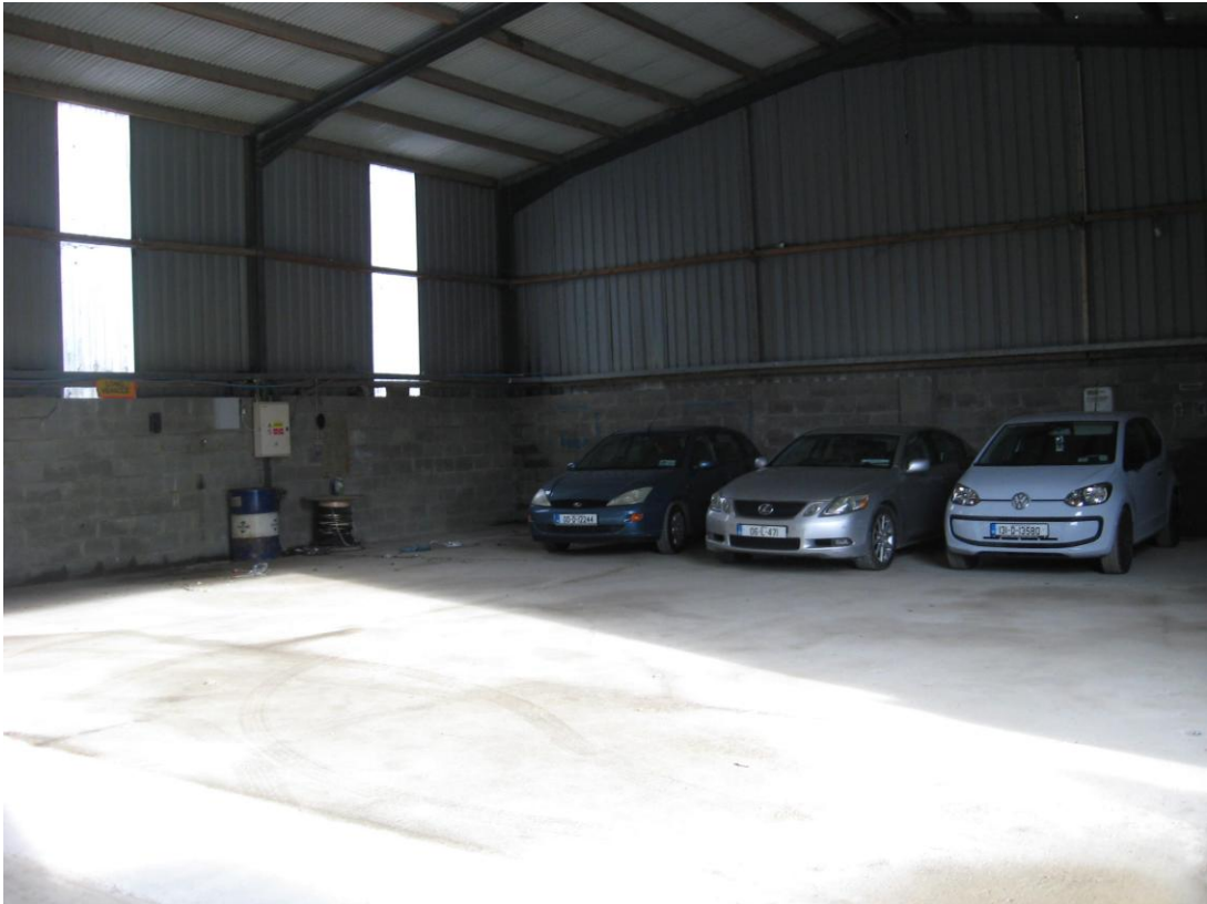
(Sample view of the interior of the 'Maintenance & Garage' Structure)
