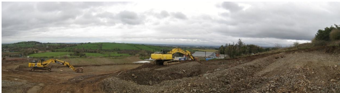
(Sample view of topsoil stripping presently underway on site)
