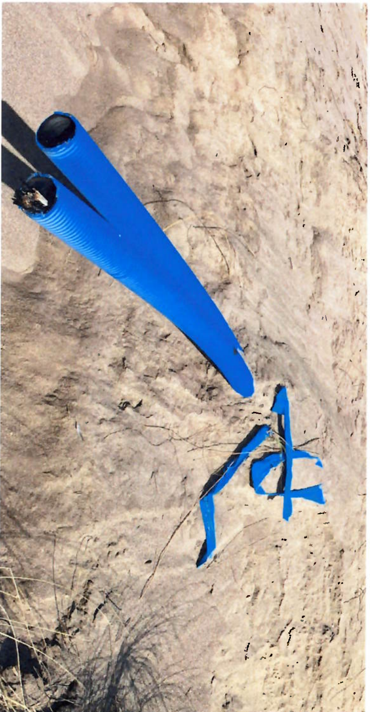
View 1 – Existing remnant of ESAT 1 cable works exposed from storm damage on dunes, looking shoreside landward to be remediated as part of the consent issued from Wexford County Council. Note – the blue duct on right contains a cut-off of the telecoms cable visible
