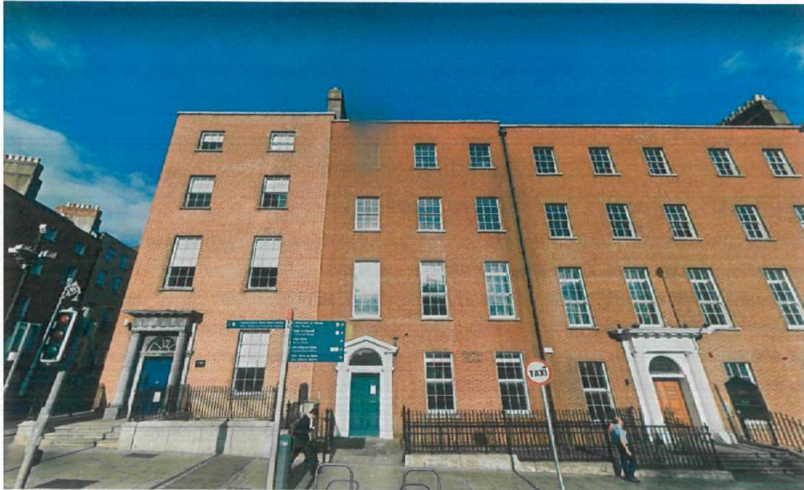
Figure 4. No. 14-16 Parnell Square East (right to left)
