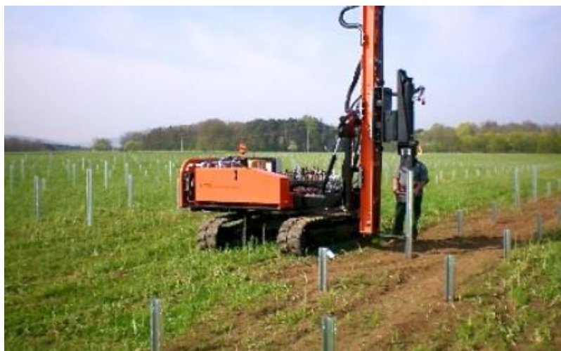
Figure 9 – Typical Low Ground Pressure Screw Pile Vehicle
