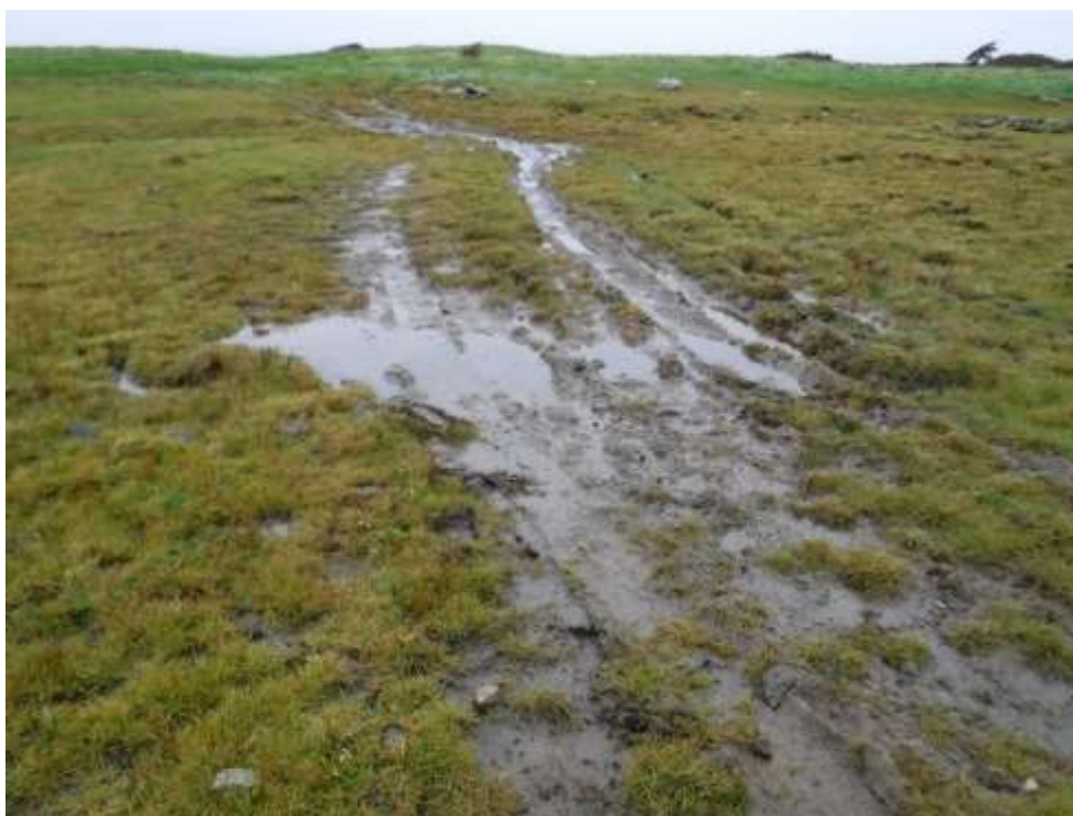
Figure 8: Damage to Salt Marsh due to tracking by farm vehicles and poaching.
