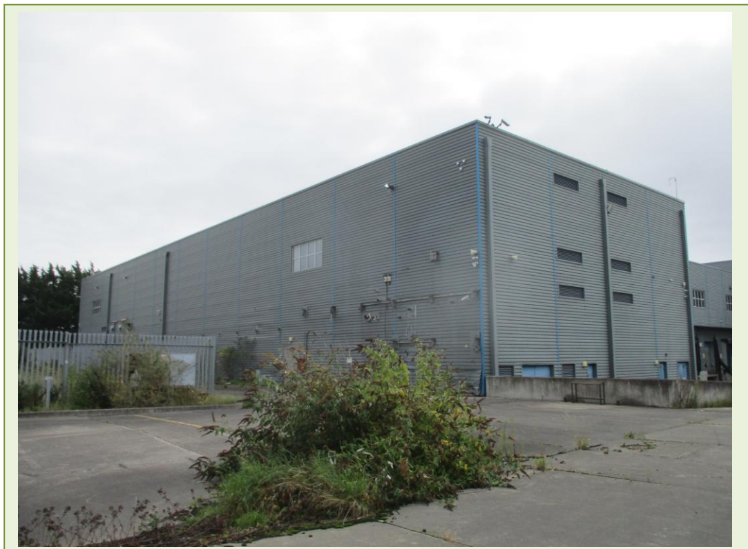
External cladding on warehouse building. No ACM's detected
