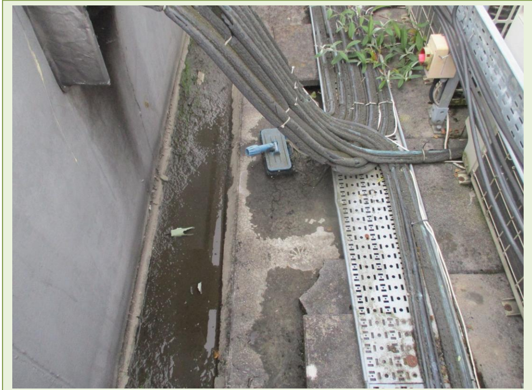
Felt on flat roof area of office block. No ACM's detected
