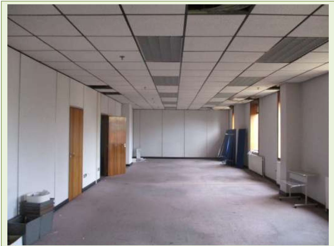
Ceiling tiles. No ACM's detected
