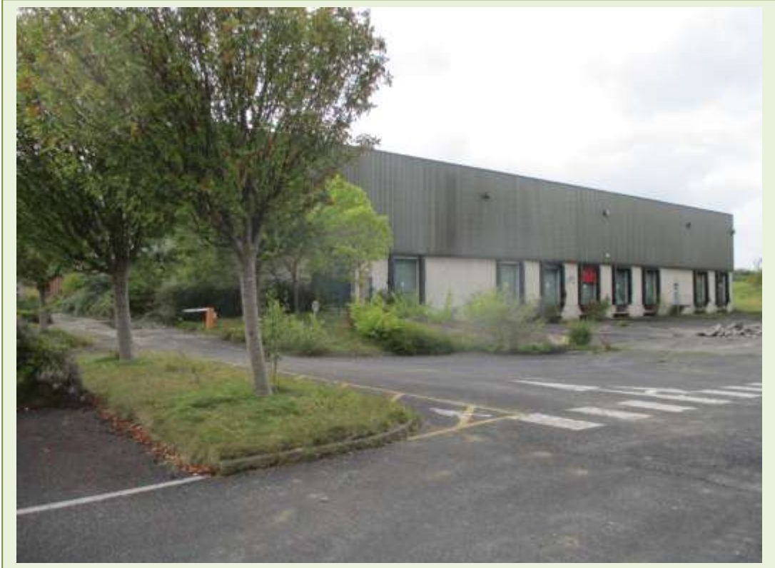
Metal cladding. No Asbestos Containing Materials (ACM's) detected
