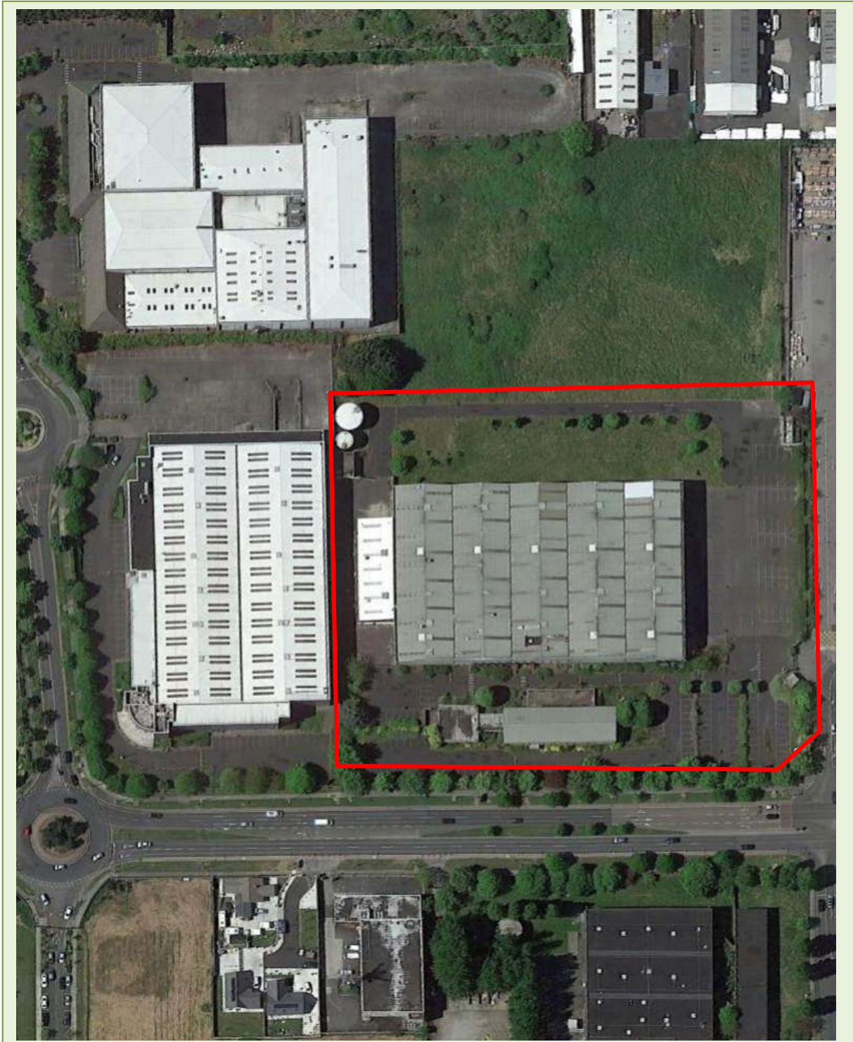
Former Uniphar Site, Belgard Road, Tallaght, Dublin 24
