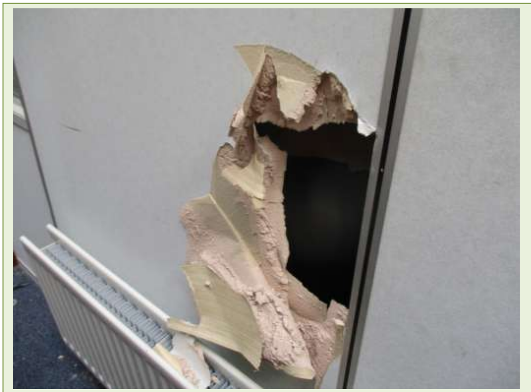
Wall panels. No ACM's detected
