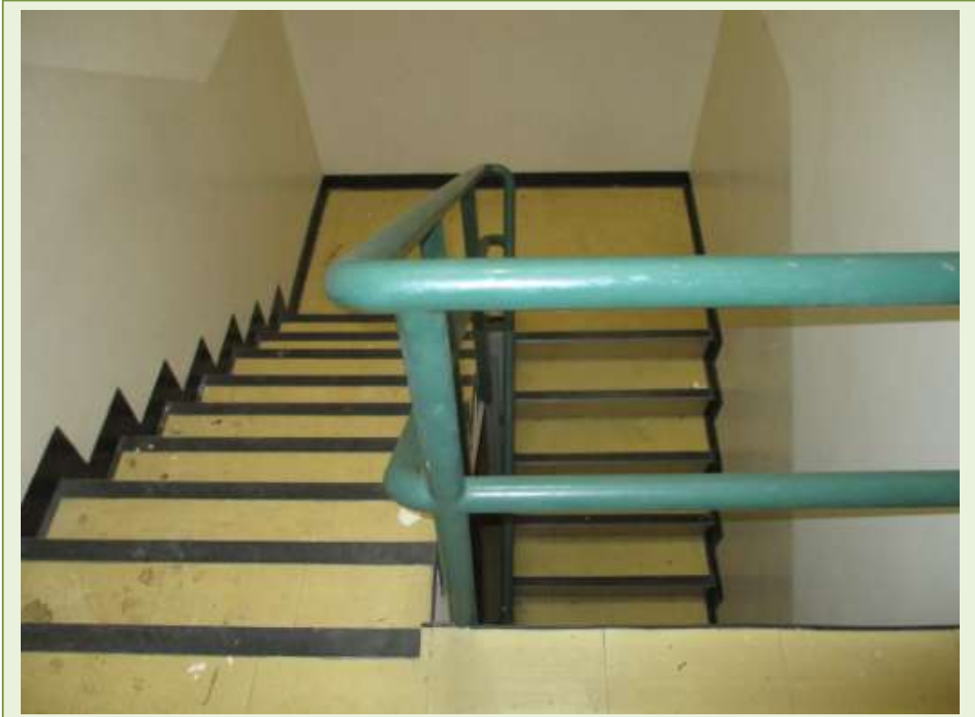
Step nosings. No ACM's detected
