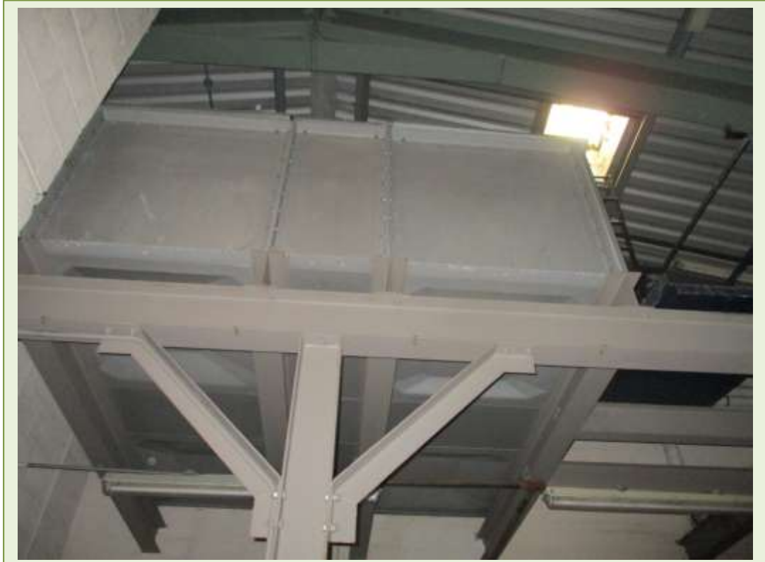
Water tank. No ACM's detected
