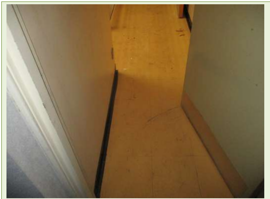
Floor tile identified in the office areas of the industrial unit
