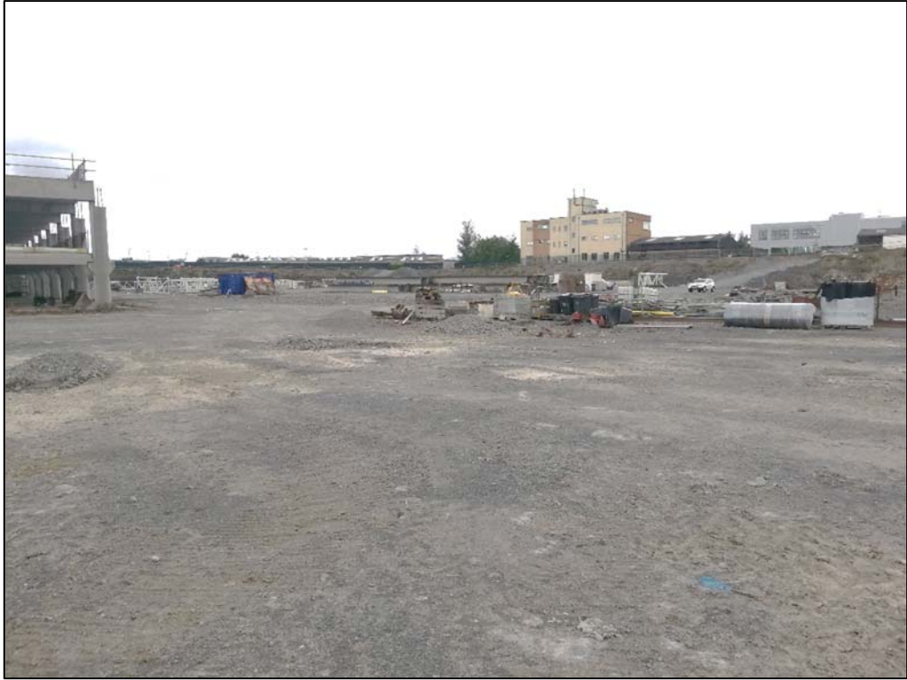
Plate 5.2 Spoil and bare ground (ED2) & existing buildings (BL3) (June 2019)
