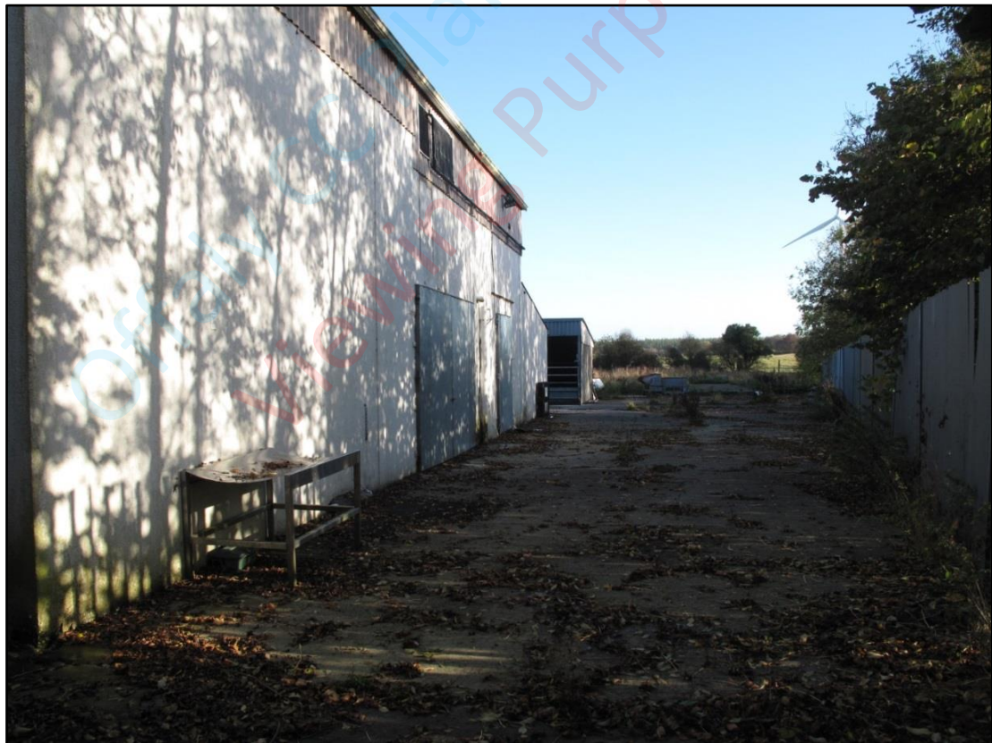
Plate 2 View to rear of site, along southeast elevation of buildings
