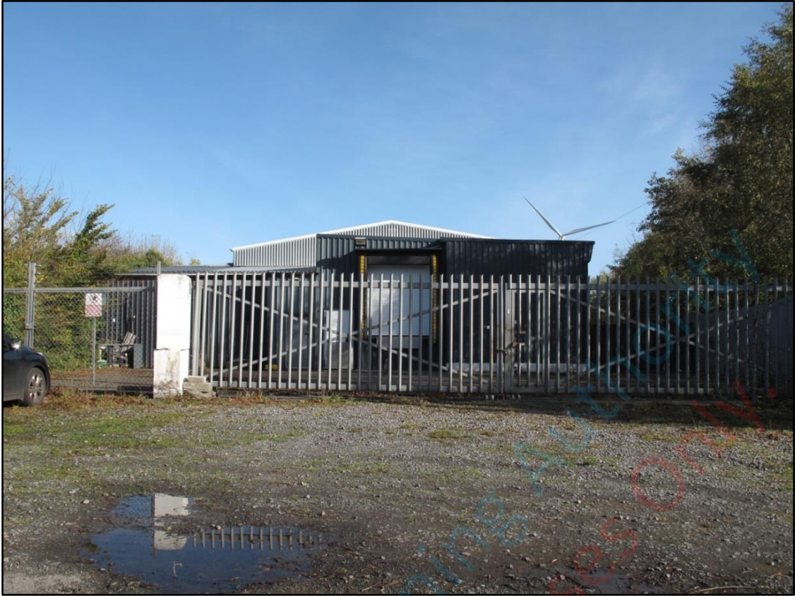
Plate 1 Front (southwest) elevation of existing abattoir buildings
