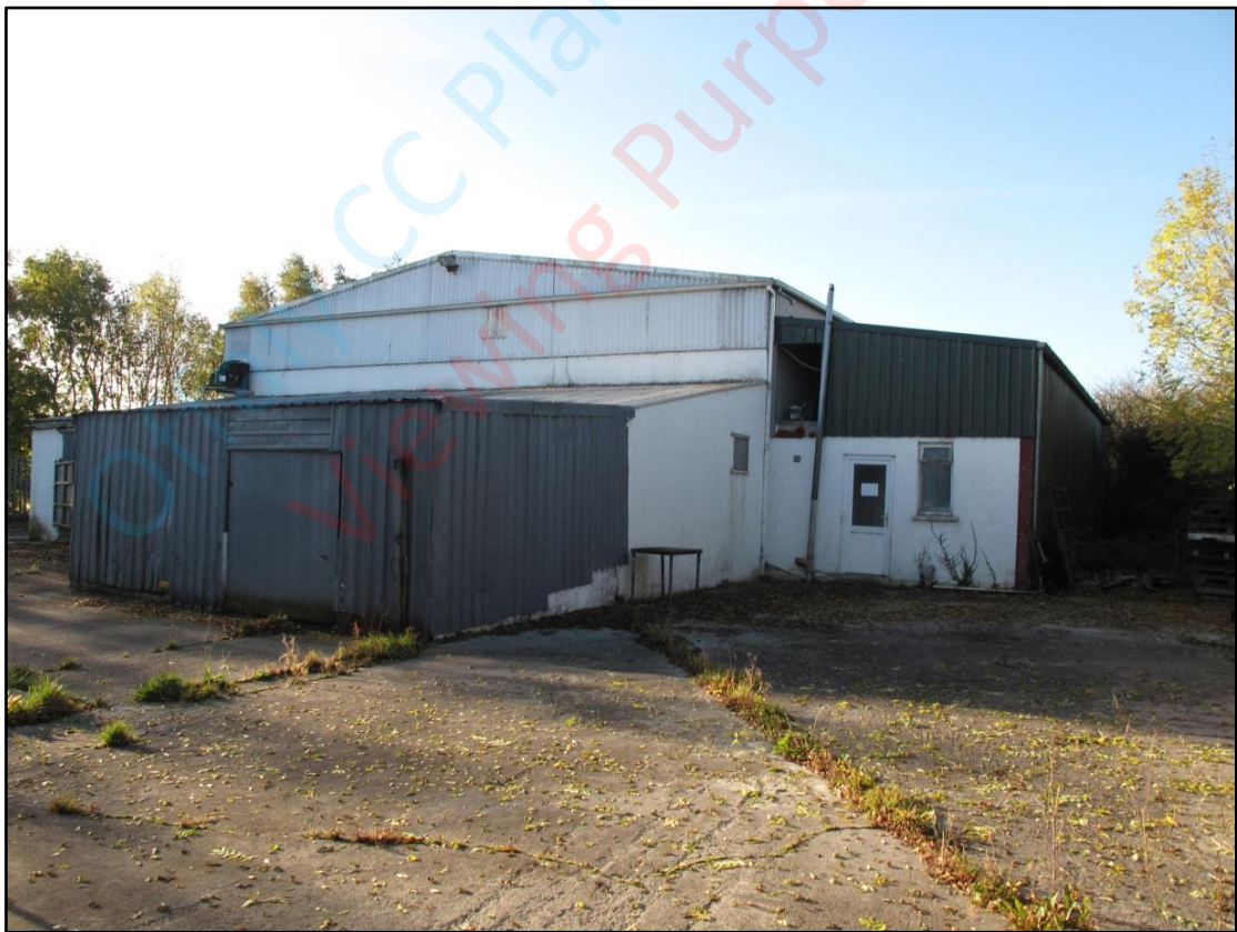
Plate 4 View to rear of existing abattoir buildings
