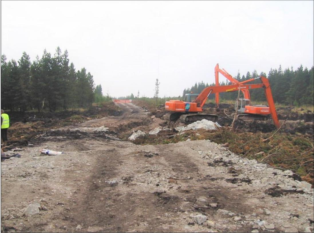
**Plate 16-1 - Excavation at Turbine T68 at the time of the slide**
