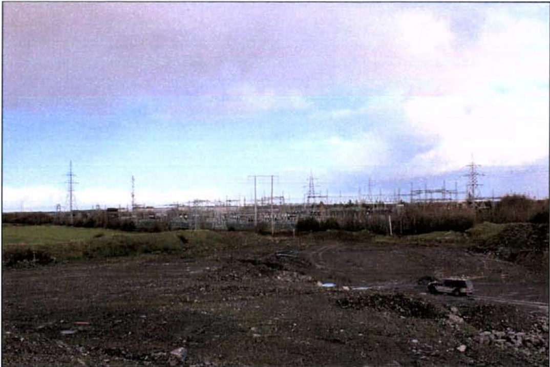
Plate 10.3 Surrounding landscape showing the existing battery storage unit on the northeast corner of the site.
