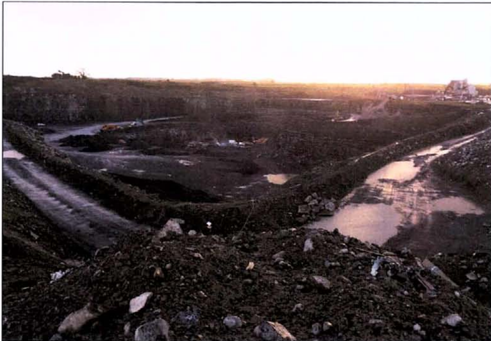
Plate 5.1: View of the active quarry, mapped as Active quarries and mines (ED4) with areas of spoil and Bare ground (ED2) and Recolonising bare ground (ED3) within the east of the site.
