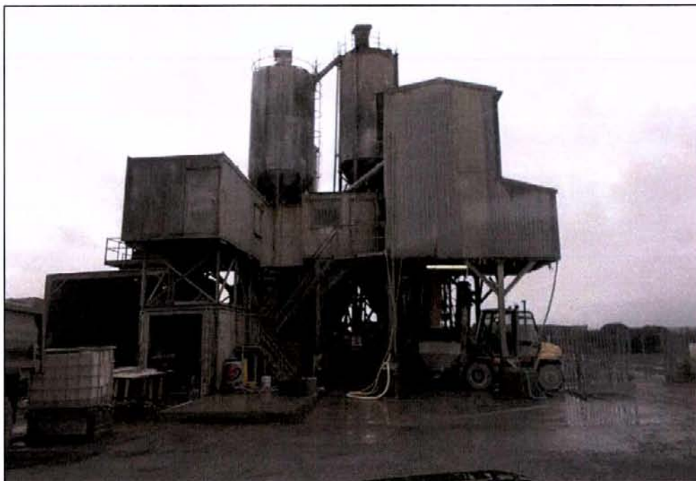
Plate 5.8 – Example of buildings and artificial surfaces (BL3) within the north-west of the site.
