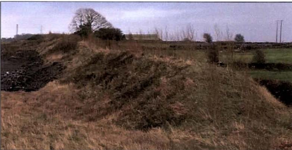
Plate 5.6: Example of planted treeline on vegetated berm along the southern site boundary.
