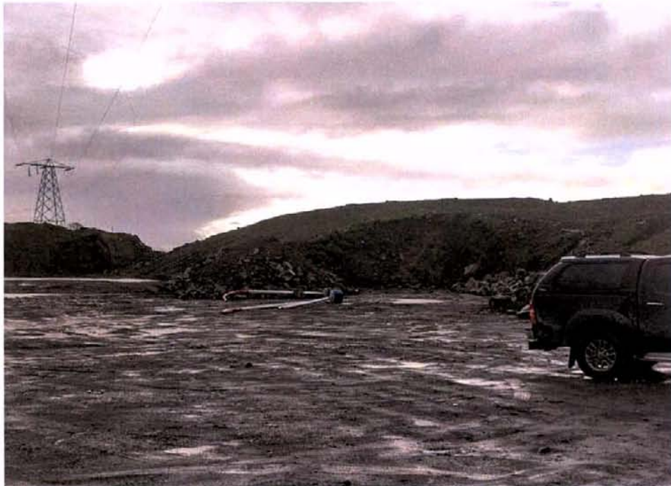
Plate 7: View from NE section of expansion area looking WSW, note area reduced to natural horizons and spoil heaps in background.
