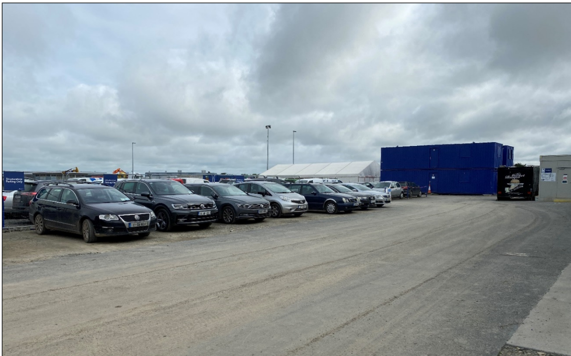
Figure 6.5 Buildings and artificial surfaces (BL3) within the Proposed Development site
