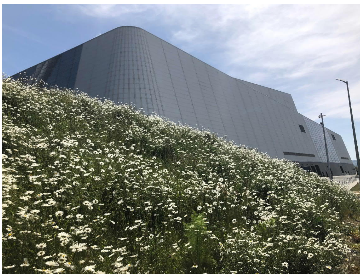
Figure 8-2 Wildflower Meadow Located at the Front of the Facility
