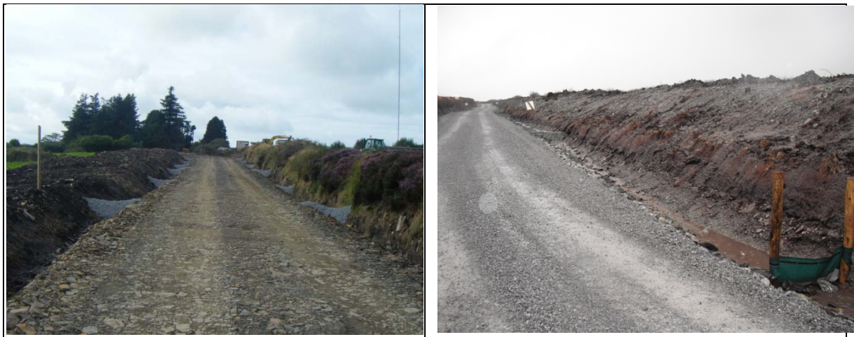
FIGURE 1 EXAMPLES OF CHECK DAMS AND EXAMPLE OF SILT FENCE USED IN CONJUNCTION WITH CHECK DAMS ALONG ROADSIDE DRAINAGE CHANNELS
