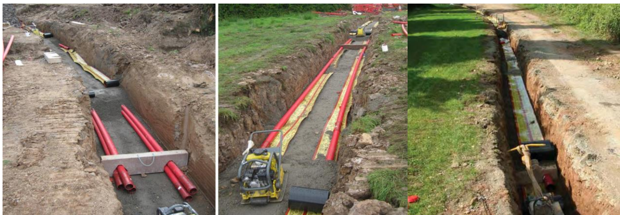
Plate 5-2: Examples of underground cable trenches
