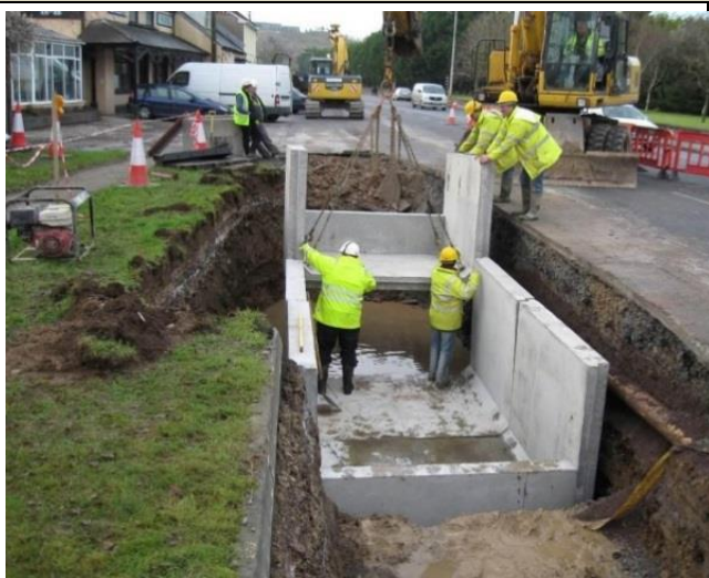
Typical joint bay under construction (pre-cast)
