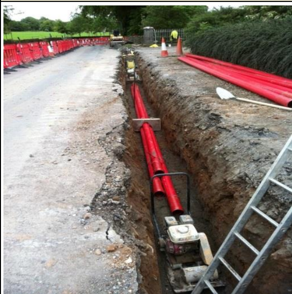
Typical 110kV Cable Trench on public roads
