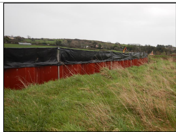
Plate 5.2: Example of visual screening used along flood defence works
