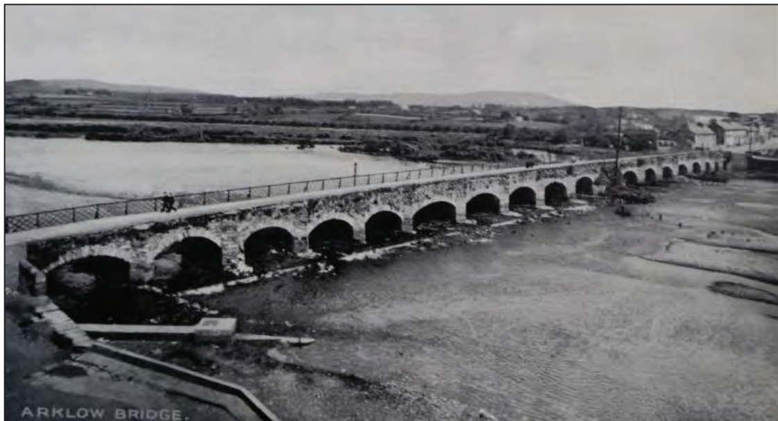
Figure 11.8: Photo of Arklow Bridge, date unknown, taken from the South Quay showing the bridge in advance of the modern interventions., showing the wrought iron pedestrian pathway and oil lamps
