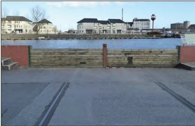
Figure 16.8 Slipway (referred to as Tyrells slip) along South Quay protected by a wooden demountable.
