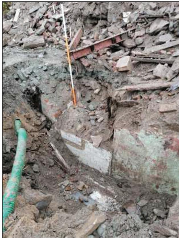
**Plate 2.4: SC3-1, detail of NE room of basement – window and Belfast sink insert**
