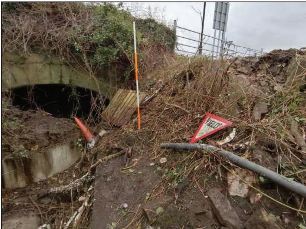
**Plate 2.6: Arched culvert and watercourse with foundation level of gable of the 1865 extension to the right**
