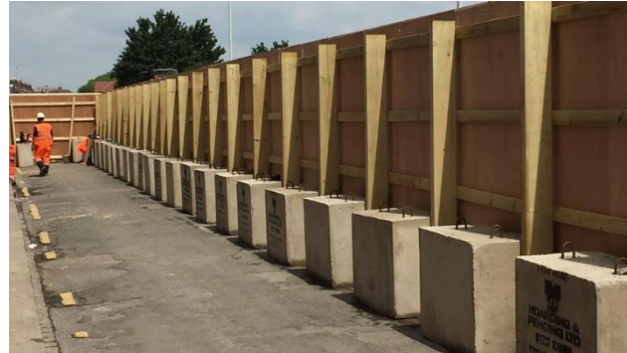
Example – Solid timber hoarding with ballast blocks
