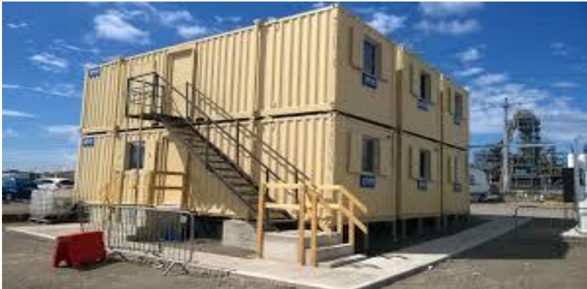
Figure 6 – Example of stacked site offices
