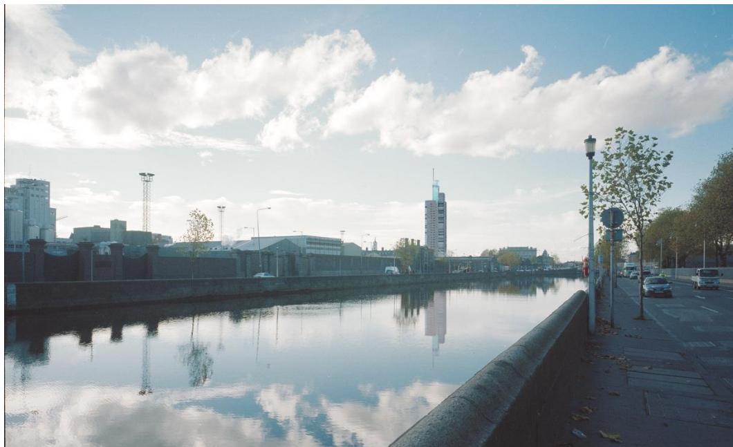
Figure 13.12: View of the proposed 32 storey residential tower which was to form part of a development on OPW lands at St John's Road / Military Road and designed by Paul Keogh Architects for the Office of Public Works. Planning approval was granted in 2005. (image ARC Consultants)
