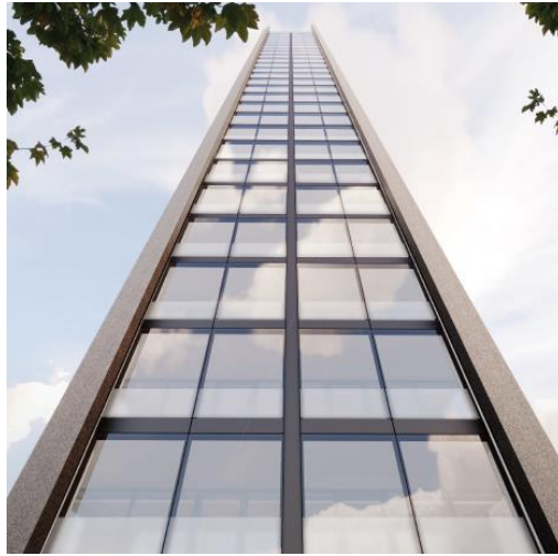
Figure 2.2: Showing the curtain wall glazing
