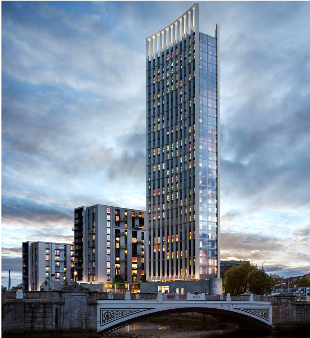
Figure 3.2: 3D Image of the proposed Block A, showing the context of the approved Blocks B and C to the rear.
