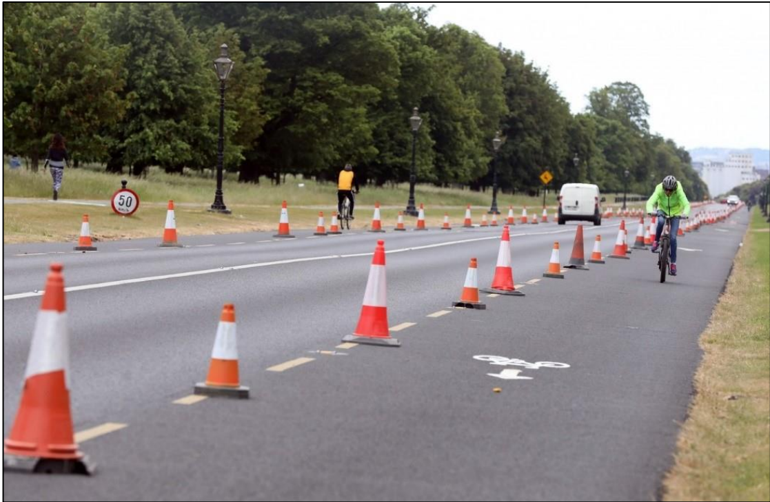
Figure 6. 4: Temporary segregated cycle lanes at Chesterfield Avenue
