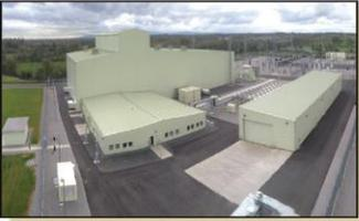
The interconnector will use High Voltage Direct Current (DC) technology, the global standard for the transfer of electricity over long distances using subsea cables. The electricity systems in Ireland and France both use Alternating Current (AC) technology, so converter stations are required at either end. The converter station is an industrial type building and outdoor compound with typical dimensions of 300 m x 150 m and a height of up to 25 m.
