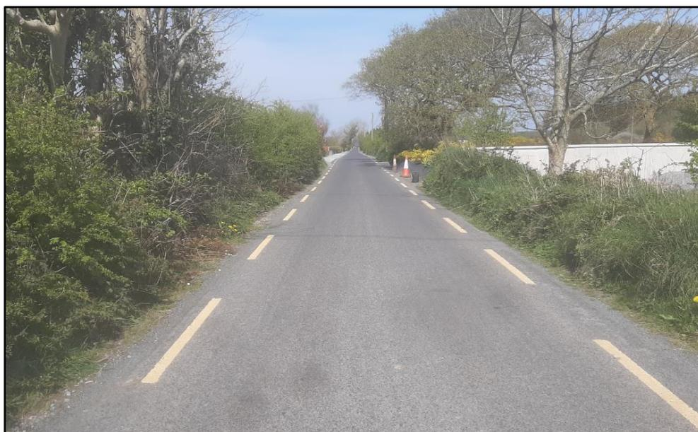
**Figure 2.5: Kilpaddoge-Knockanure 220 kV UGC project: Reinstated local public road following the laying of UGC.**
