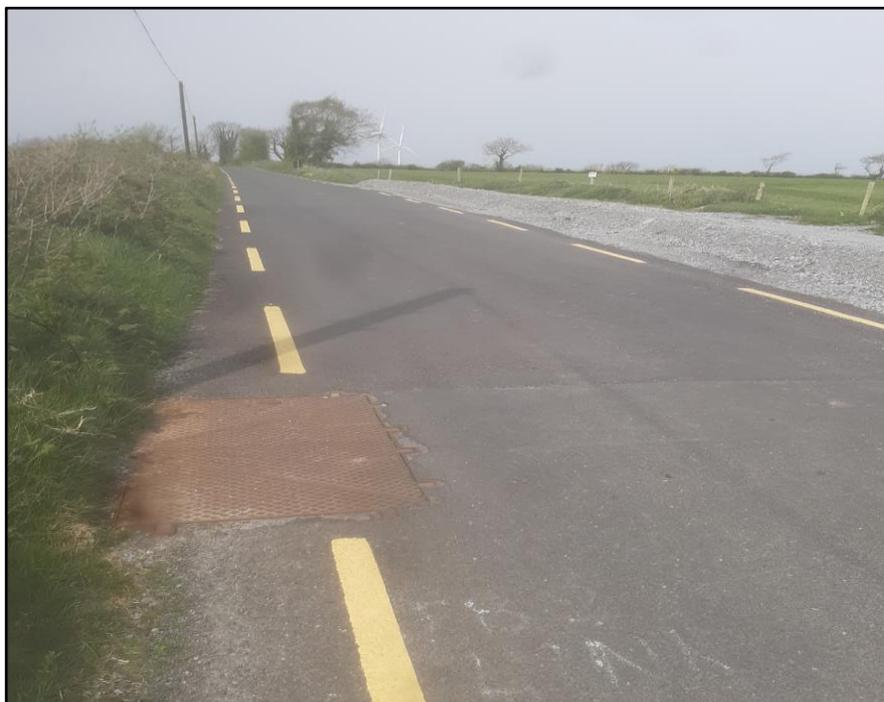
**Figure 2.4: Kilpaddoge-Knockanure 220 kV UGC project: Reinstated public road at a joint bay location (darker tarmac on road), with associated fibre optic link box (brown metal surface), and passing bay currently dormant and bermed with stone prior to jointing works at the joint bay**
