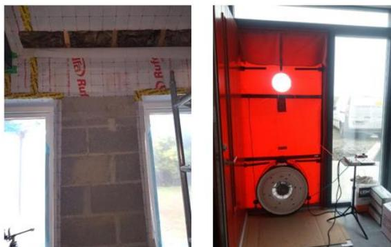
Figure 3 – Air Tightness Testing
