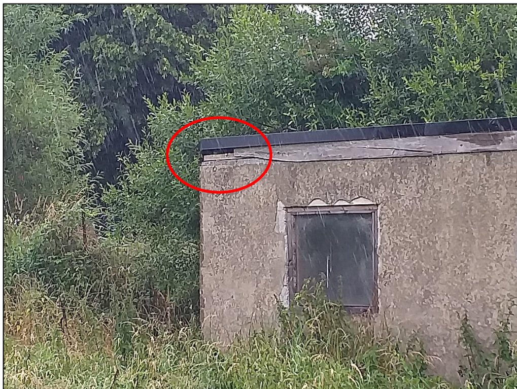
Figure 6. Old Shed/outhouse with missing part of fascia board on the northwest corner of structure
