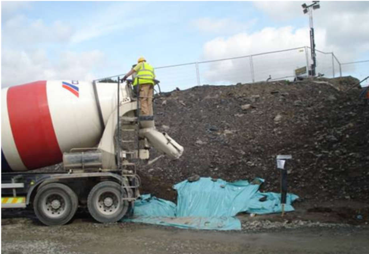
Figure 3-3 Concrete wash-out area with impermeable liner (TII)
