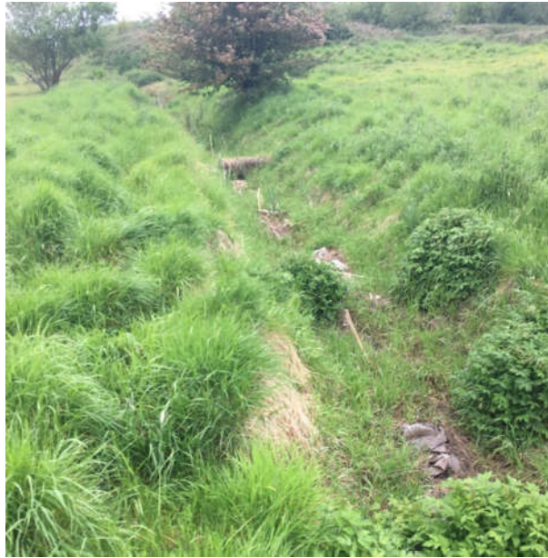
Photo 3-2: Existing drain on old racecourse to the north of SHD site
