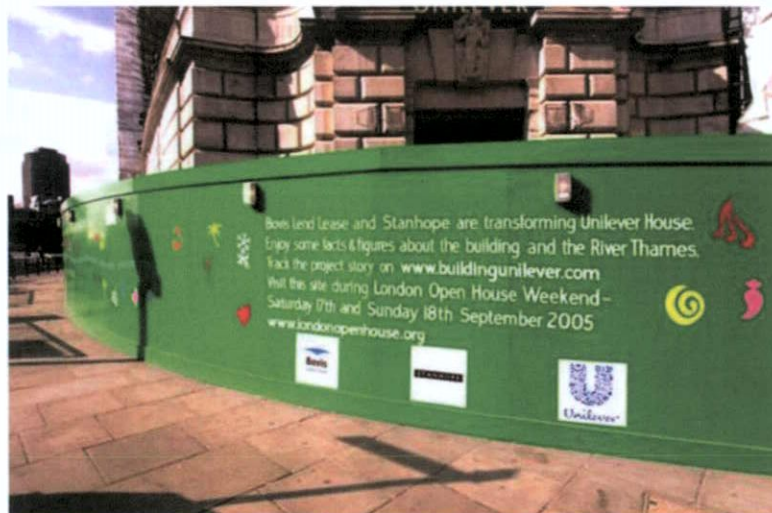
Figure 5 – Typical pavement hoarding with street lighting
