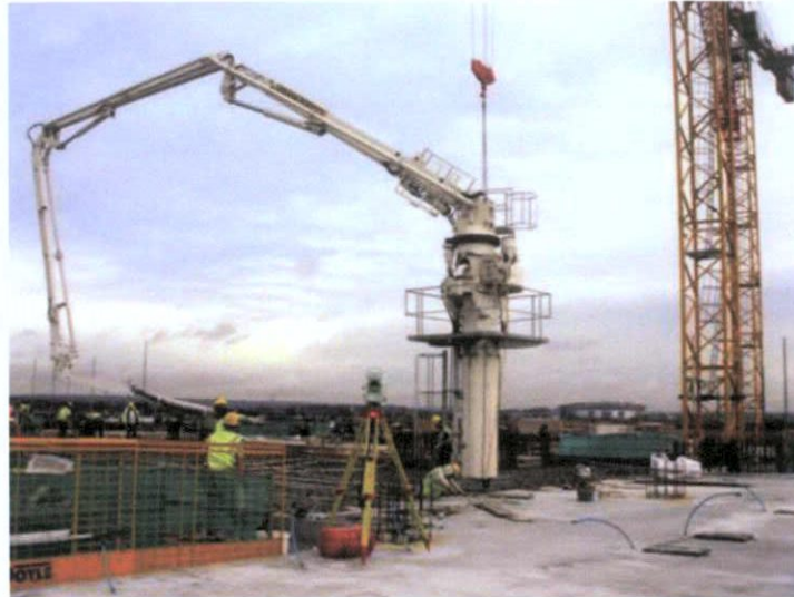
Figure 15 - Typical Concrete Placement
