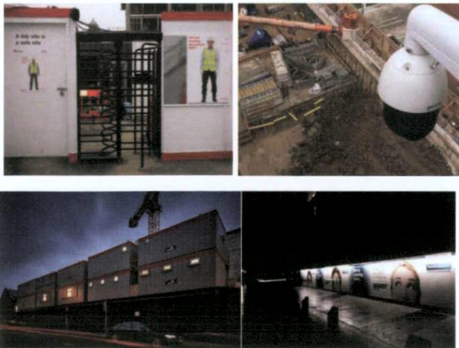
Figure 9 _Typical Site Security Measures
