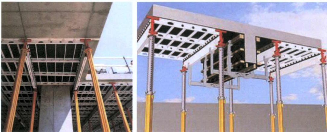
Figure 14 - Typical RC Formwork (Skydeck)
