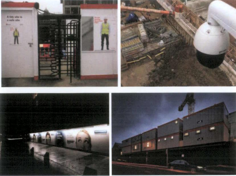
Figure 9 – Typical Site Security Measures
