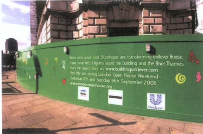
Figure 5 – Typical pavement hoarding with street lighting
