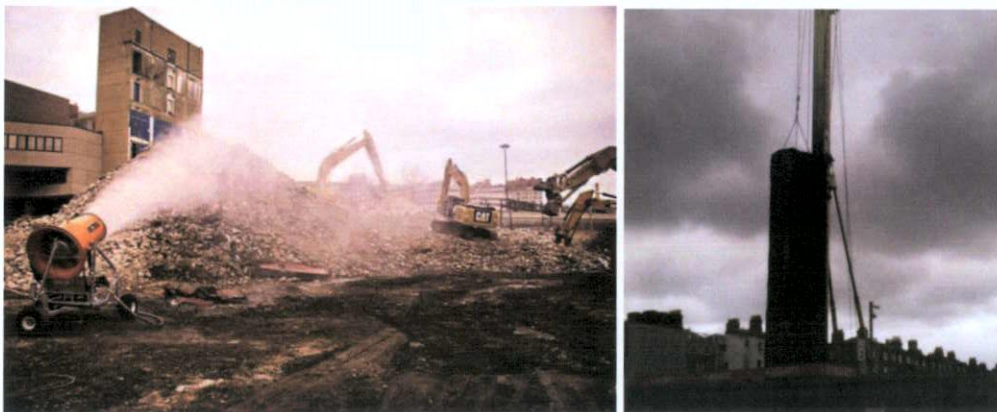
Figure 27 – Typical Dust Mitigation Measures
