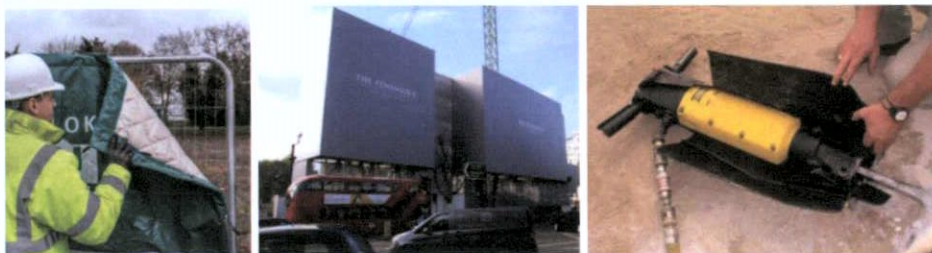
Figure 26 – Typical Noise Mitigation Measures
