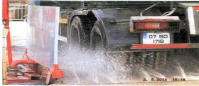
Figure 8 – Typical Wheel Washing Facility
