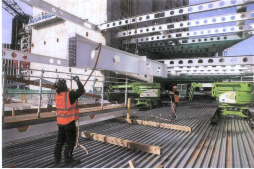
Figure 16 – Typical Steel Frame Erection
