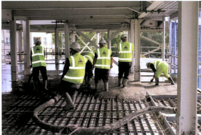
Figure 17 – Typical Concrete Pour on Metal Decking
