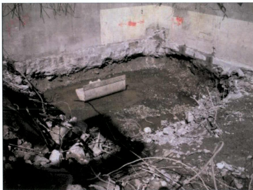
Figure 27 Trench 4, temporary crane base
