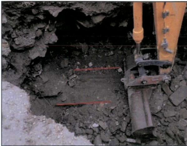
Figure 60 The structure from the north
