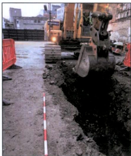
Figure 45 Trench 1, from the east
