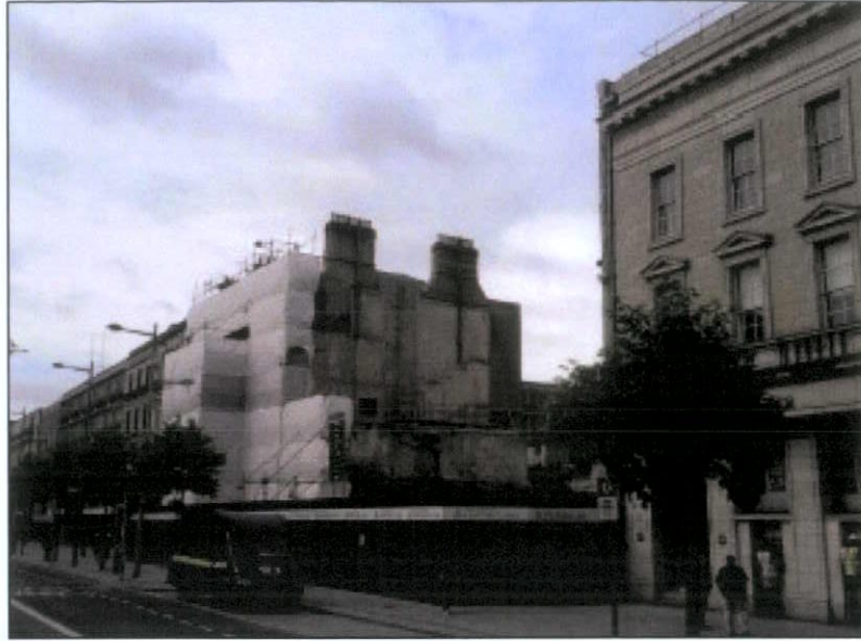
Figure 21 After the demolition of the Royal Dublin hotel
