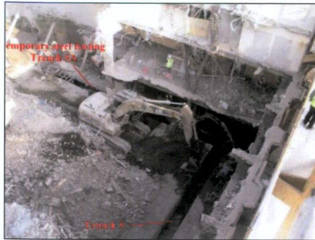
Figure 23 Overview of steel footing trench
