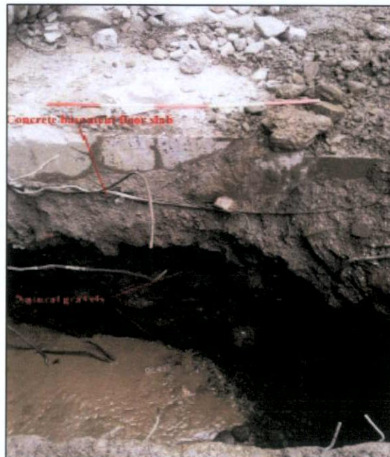
Figure 25 Trench B, concrete and natural gravels
