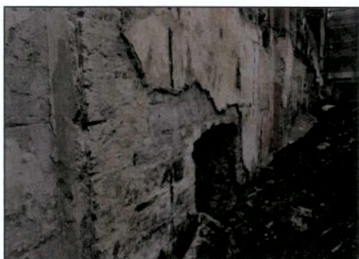
Figure 76 Projecting chimney breast
