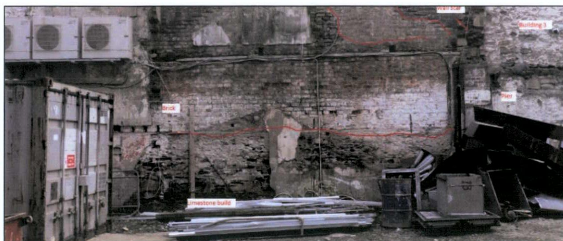
Figure 90 Boundary wall between No. 51 and 52 (from the north)
