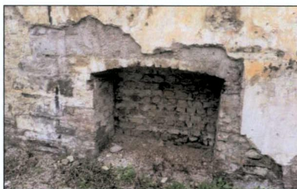
Figure 77 The fireplace in Room 2: type 3 brick
