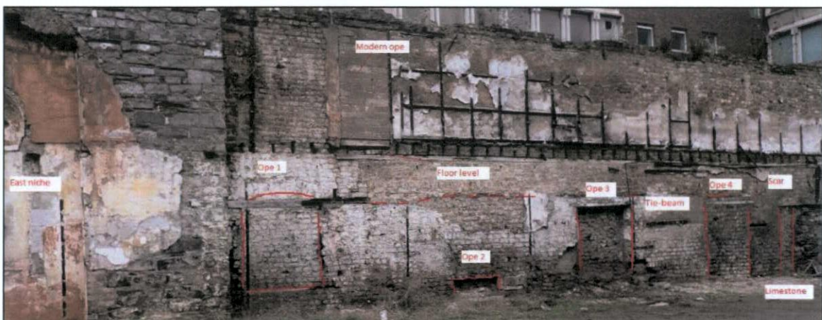
Figure 83 Building 3, from the west
