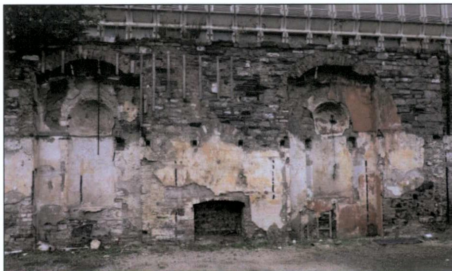
Figure 74 Building 2, from the south
