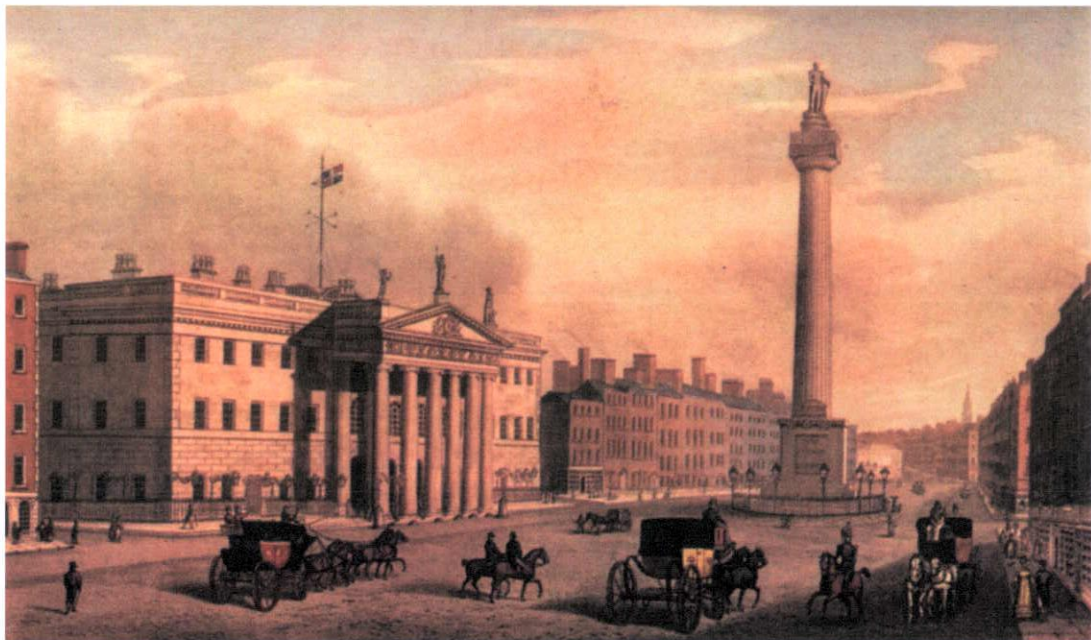
Figure 12.3: View of Sackville Street with the GOP and Nelson's Pillar by Brocas c. 1820.
