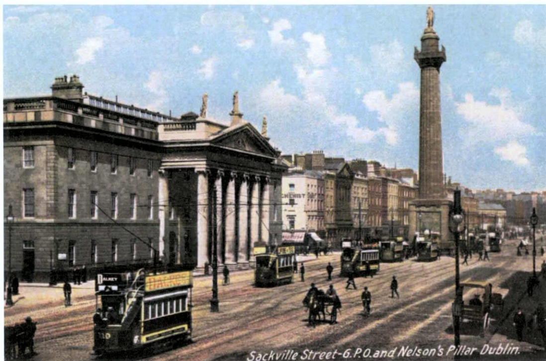
Figure 12.8: Post Card view of the centre of Sackville Street c. 1900. The GPO has long glazed rooflights above the cornice and balustrade. The Royal Coat of Arms is seen in the tympanum.
