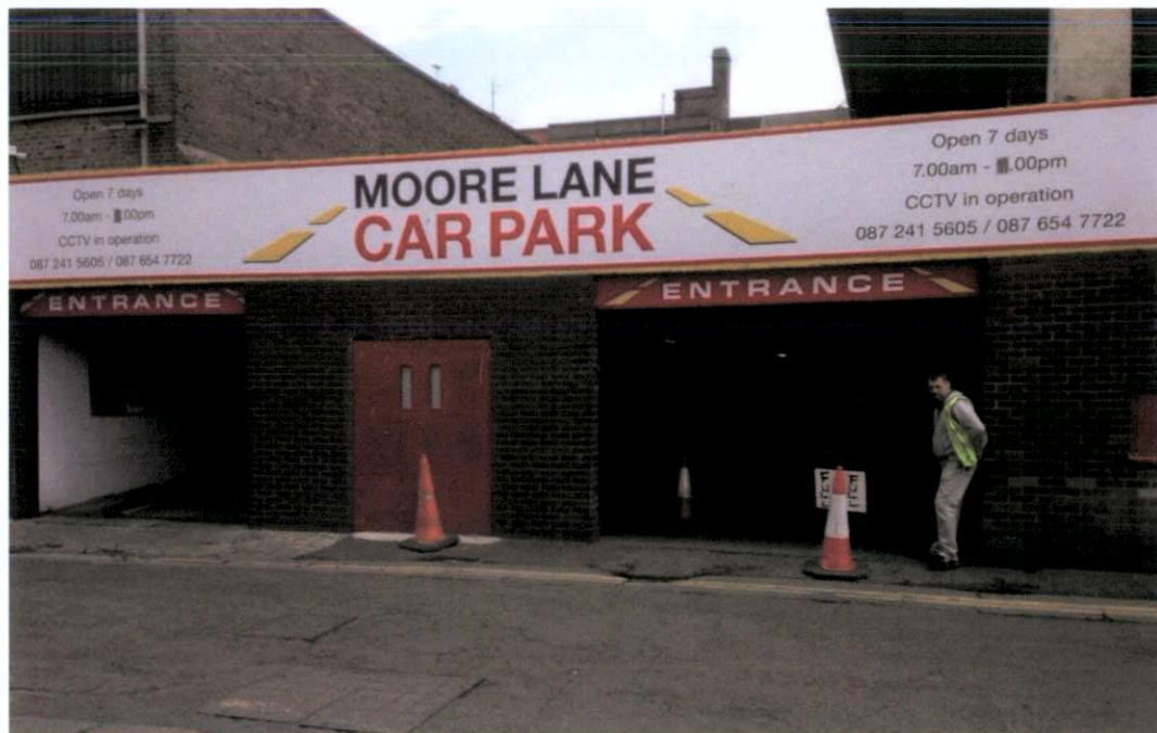
Figure 13.4: Entrance to Moore Lane Car Park.
