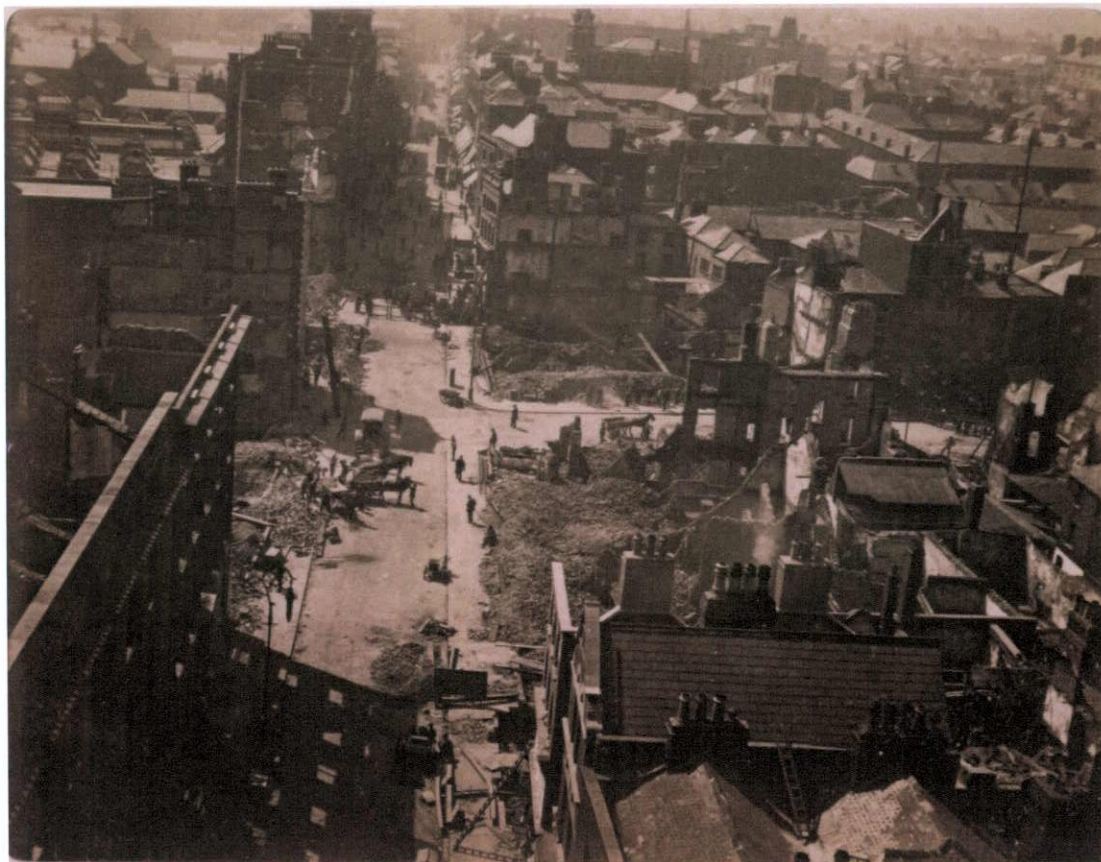
Plate 15.3.8: Photograph from the top of Nelson's Pillar showing the destruction of the urban block of Site3 after the 1916 Rising. The terrace on Moore Street is demolished as far as the site of 34 Henry Street where the gable wall survives. The rear walls of Moore Street terrace and three chimneystacks are standing. (Digital Repository of Ireland)
