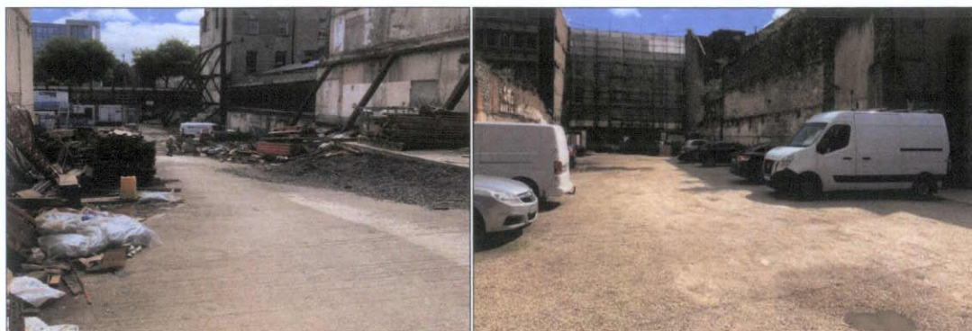
Figure 16.16: Nos. 40 – 41 O'Connell Street (left) and Nos. 50 – 51 O'Connell Street (right).
