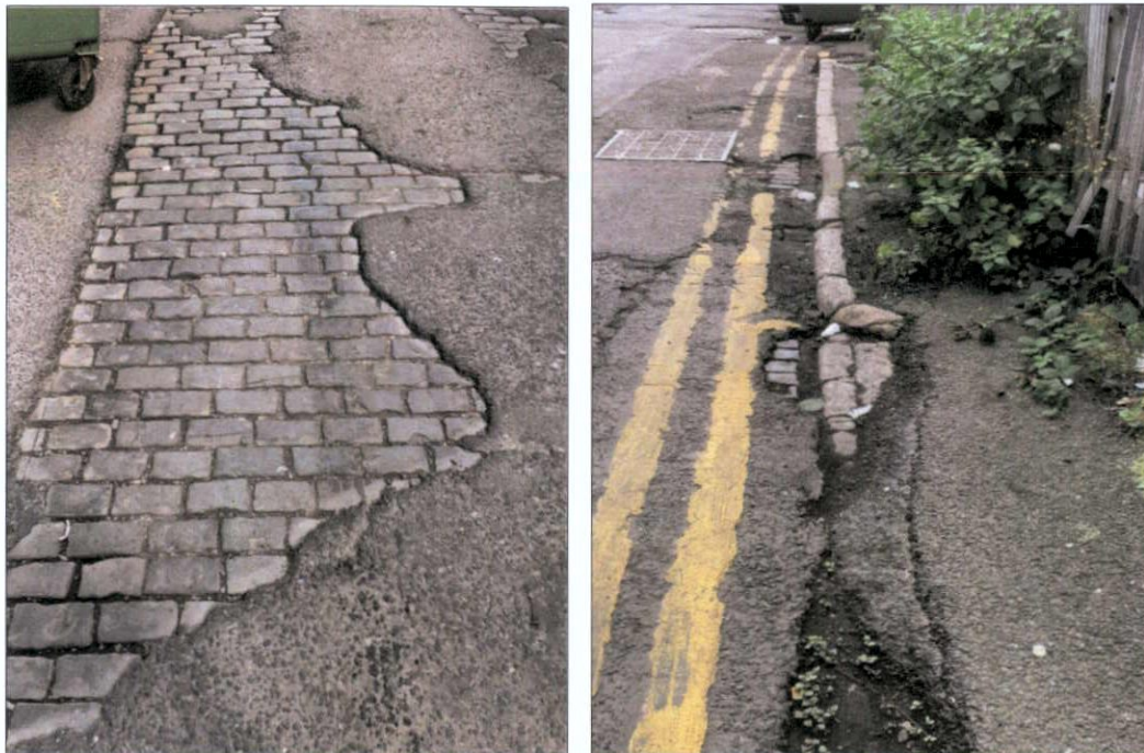
Figure 16.24: Stone paving in-situ (left) and Granite paving in-situ (right).
