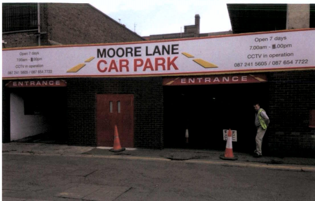
Figure 13.4: Entrance to Moore Lane Car Park.
