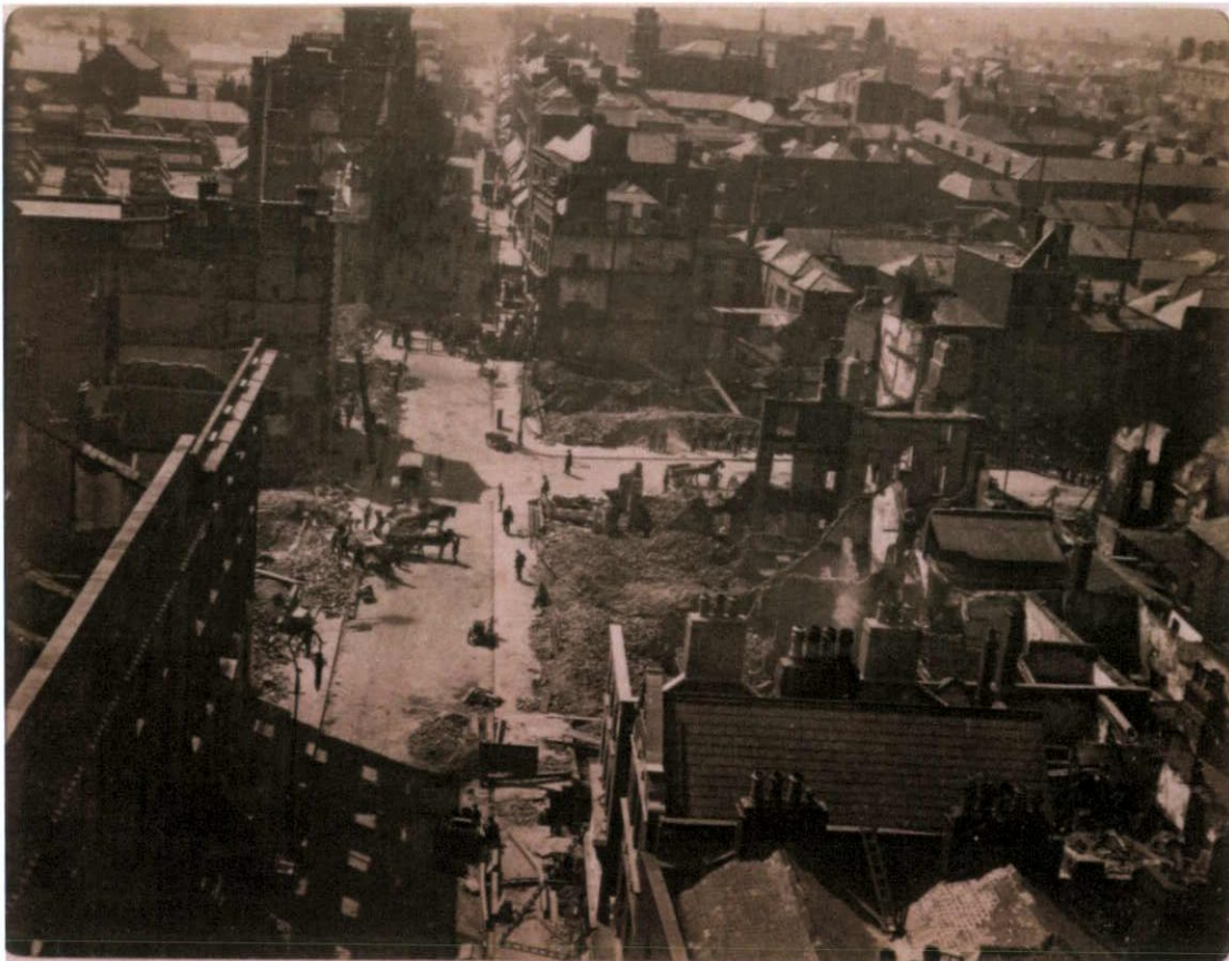
Plate 15.3.8: Photograph from the top of Nelson's Pillar showing the destruction of the urban block of Site3 after the 1916 Rising. The terrace on Moore Street is demolished as far as the site of 34 Henry Street where the gable wall survives. The rear walls of Moore Street terrace and three chimneystacks are standing. (Digital Repository of Ireland)
