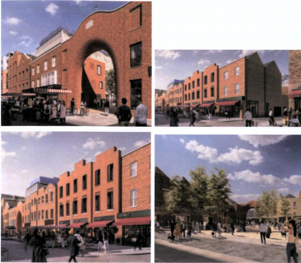
Figures 15.4.7- 15.4.10: General images of the operational stage of the Site 4 development.
