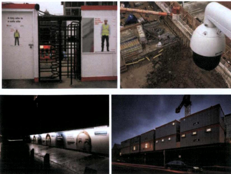
Figure 8 – Typical Site Security Measures
