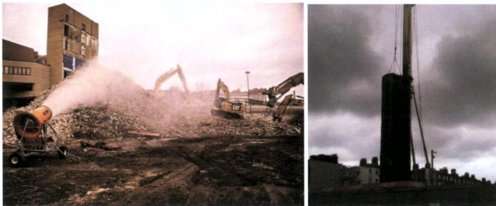
Figure 16 – Typical Dust Mitigation Measures
