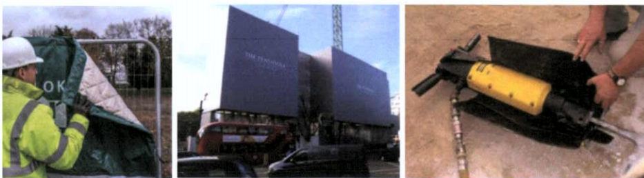
Figure 15 – Typical Noise Mitigation Measures
